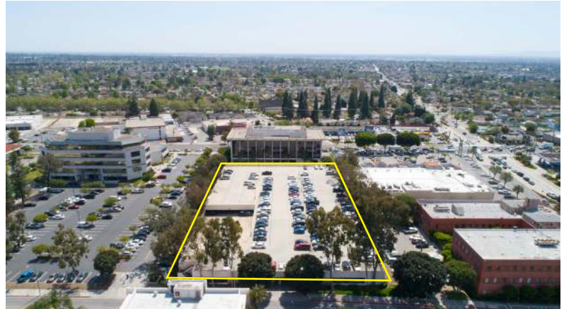
Abundant Parking Within Parking Structure
